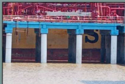
Liquid Cargo Jetty -Cathodic Protection of RCC Piles combining advance pile encapsulation using interlocking jackets
