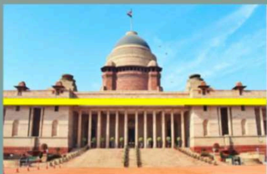
Rashtrapati Bhavan Presidential Palace ACI 2022 award winning project utilizing innovative solution for corrosion problem
